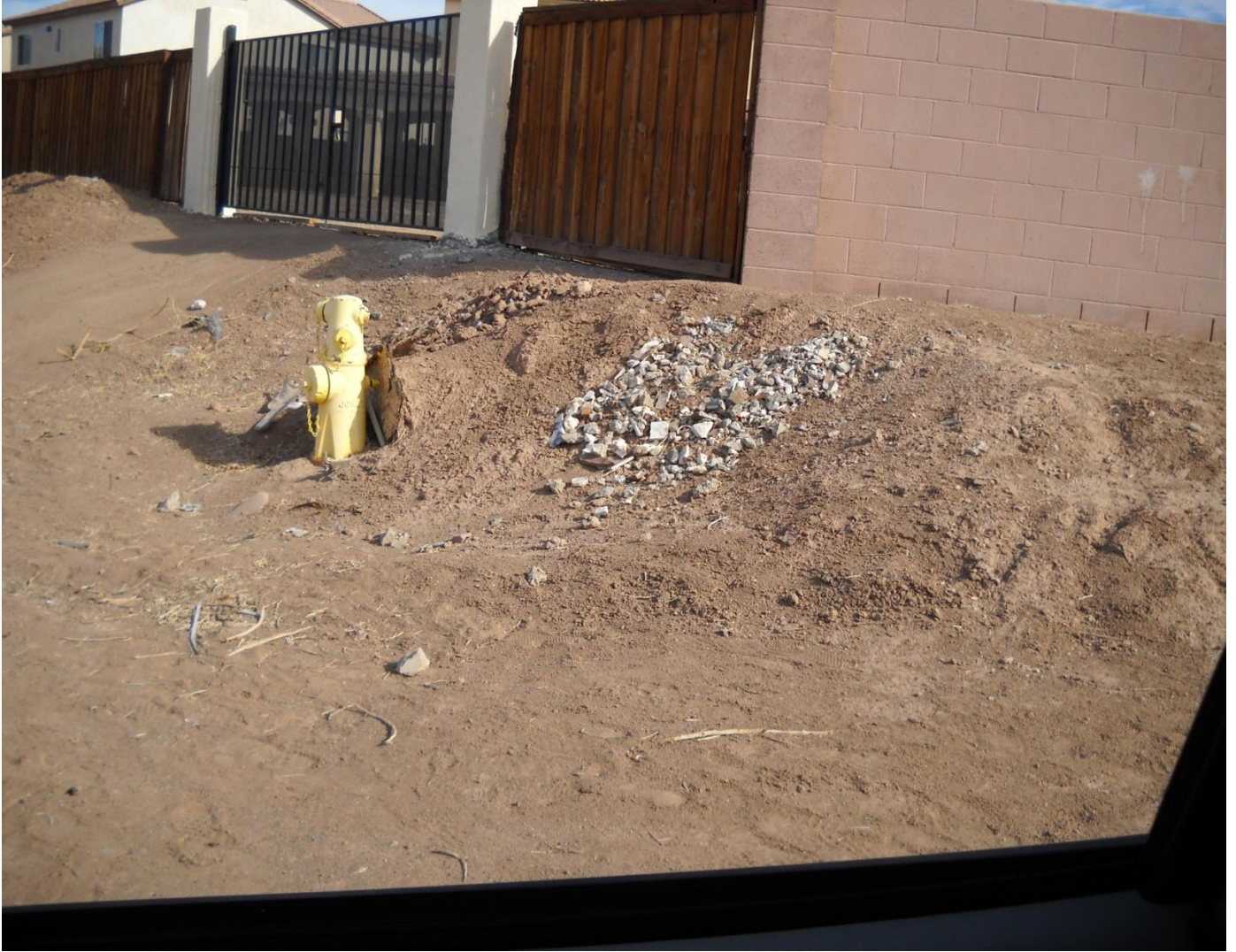
Partly blocked fire hydrant
